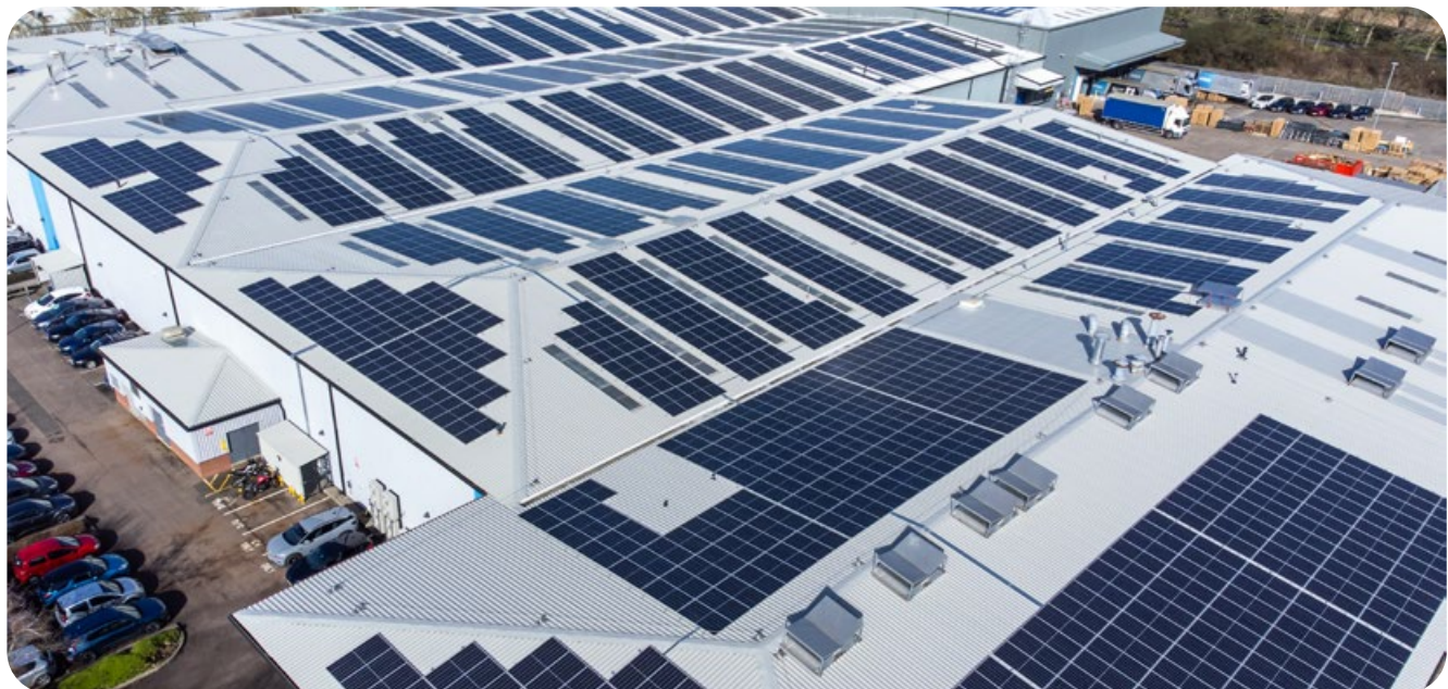
Image: Solar photovoltaic (PV) units on the roof of Thorlux's manufacturing facility
